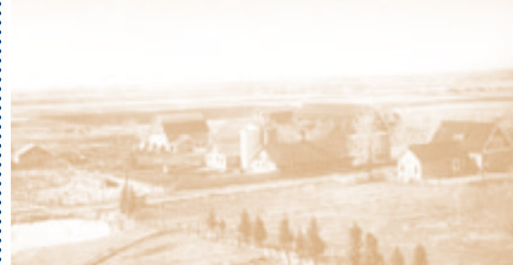
Research and teaching farm at South 3rd Avenue and Lincoln Street.
