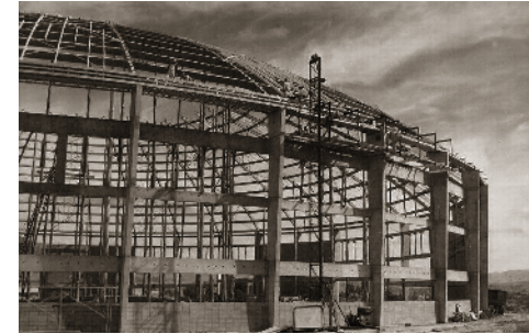
Fieldhouse dome under construction; completed in 1957 (Bozeman, MT Architect Oswald Berg).
